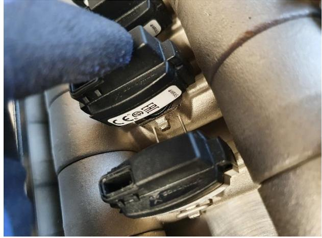
8. When the sensor is placed vertically, it can be pushed down into the piping
